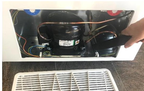
Figure 5 – Cleaning of the compressor room
